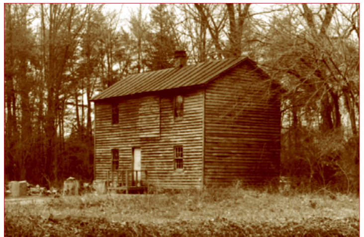
BELOW: Located near the southwest intersection of Dyson Road and Missouri Avenue, the tenant house at Ferndale Farm was a two-story, four-room, wood-frame dwelling with clapboard siding set on wood pilings. Windows were six-over-six in configuration and the house had a central chimney and standing-seam metal roof. Photo c. 1987, courtesy of Franklin A. Robinson, Jr.
