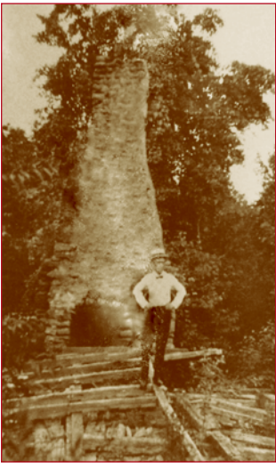
ABOVE: The much-taller chimney c. 1925, before it was modified
